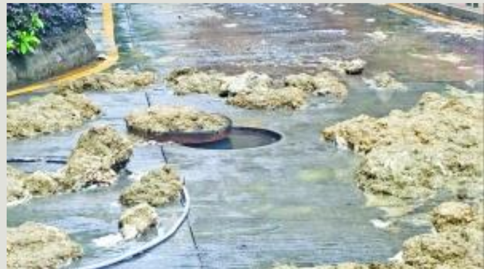
Blockage of public sewers due to improper cleaning of grease interceptors ( Rua do Rebanho )
