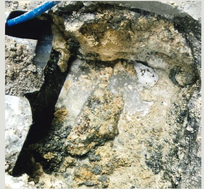
Blockage of public sewers due to improper cleaning of grease interceptors ( Rua do Rebanho )
