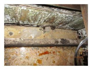
➤ The grease or water level has reached the top and the water outlet cannot be seen, showing that the grease interceptor has lost its grease separation function or the sewer has been clogged.
